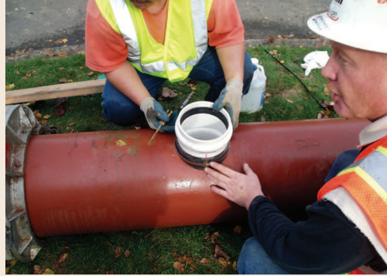
NCPI provided field training for contractors on tapping techniques for VCP.
